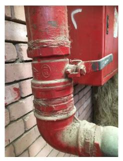
Figure 11. Flax fibre used in plumbing at Motaz Elkholy warehouse in Egypt
