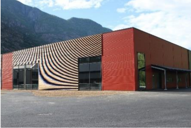
Figure 47: New packing house and retail supply outlet built by farmer cooperative adds value to farmer-members (Photo Credit: Amy Cronin)
