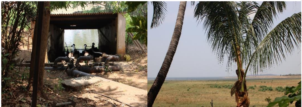
Figure 27: Irrigation pipes (left) when first installed at the edge of a lake which is now (right) 1.5 kilometres away, due to damming of the Zambezi river (Photo Credit: Amy Cronin)
